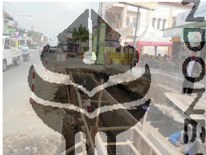
**Gambar 3. 1 Saluran Drainase Beton Konvensional**
