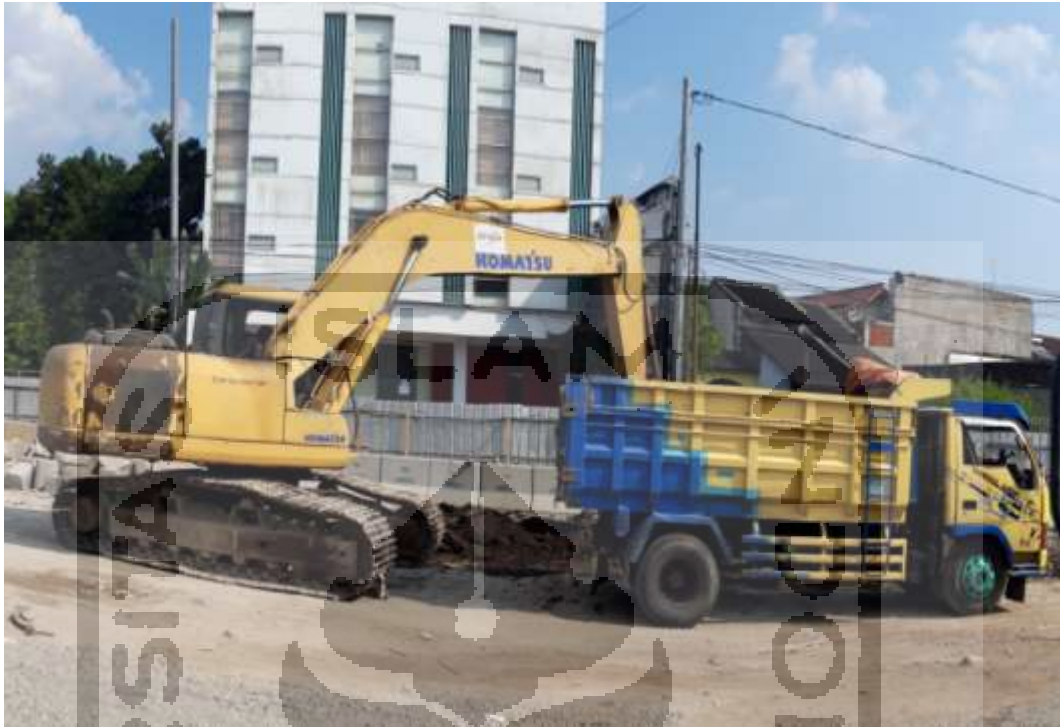
Gambar L-5. 3 Excavator Komatsu PC 200-8
