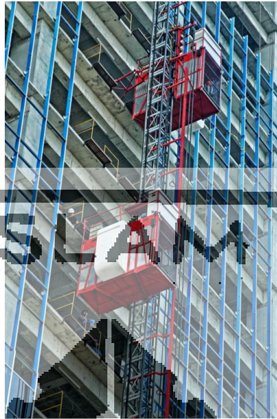
Gambar 3.4 Passenger Hoist 2 kabin (Sumber : dwijayatek-adigemilang (2019))
