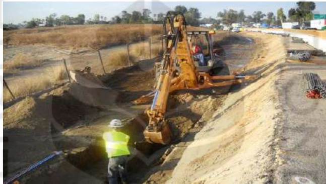
Gambar 3.12 Pekerjaan Galian Tanah Soil Nailing
