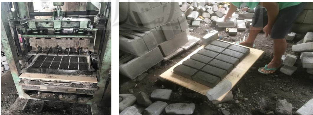
Gambar 3. 4 Proses Pencetakan Paving Block
