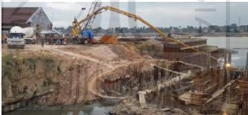
**Gambar 5.25 Concrete Pump**
