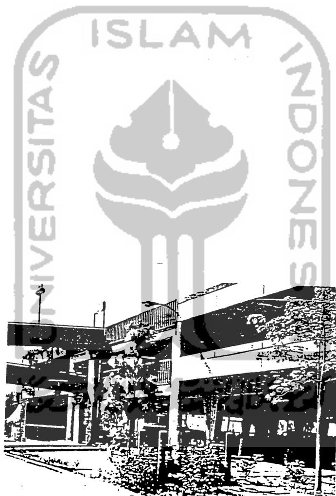
2-31 This parking structure combines precast and poured in place concrete construction. Pedestrian skyways lead to the retail portion of the complex.
