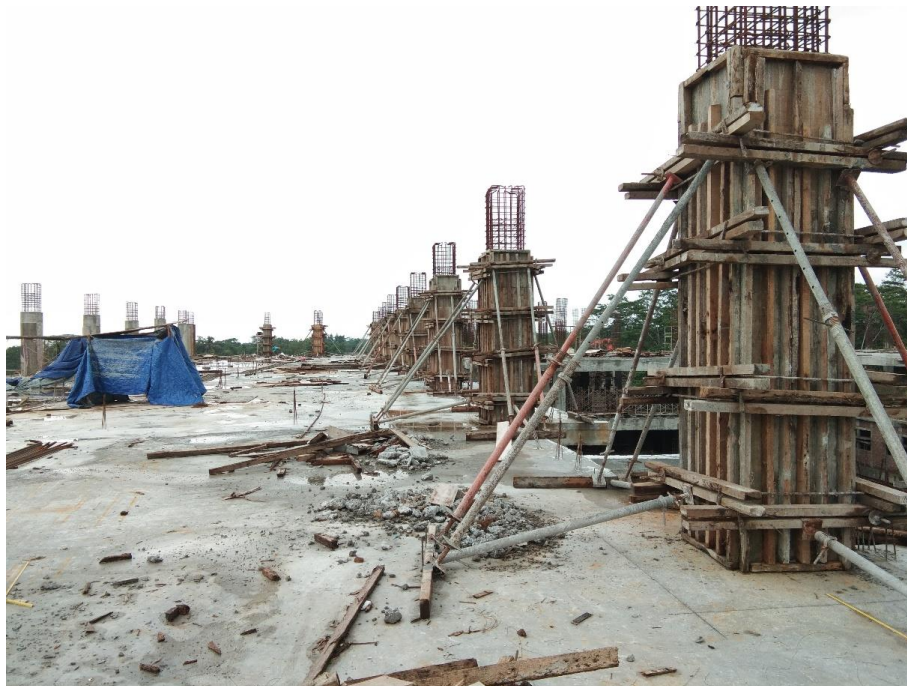
Gambar L-2.8 Bekisting Terpasang
