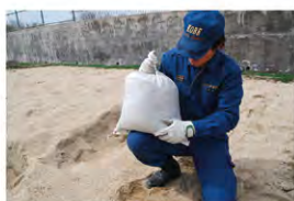
Place the sandbag on the lap.
