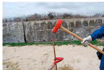
How to Drive in a Stake
