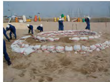
Sandbag Stacking in a “Stepped Pot” Shape
