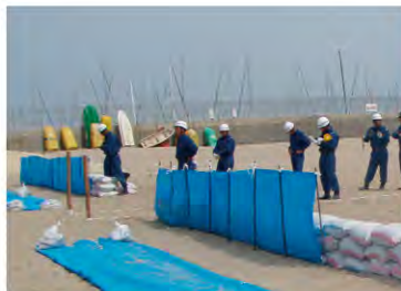
Sandbag Stacking with a Tarpaulin Wall
