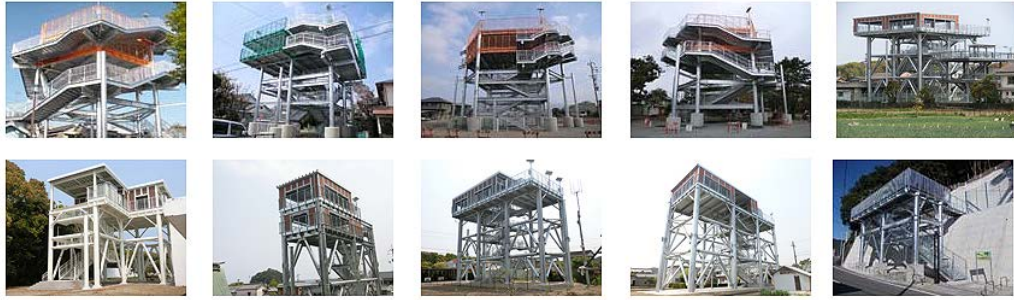
Gambar 11. Tsunami Evacuation Tower – Fujiwara Industry Co., Ltd. http://japan-product.com/ads/fujiwara-industry-co/fujiwara_industry-tsunami_evacuation_towers/
