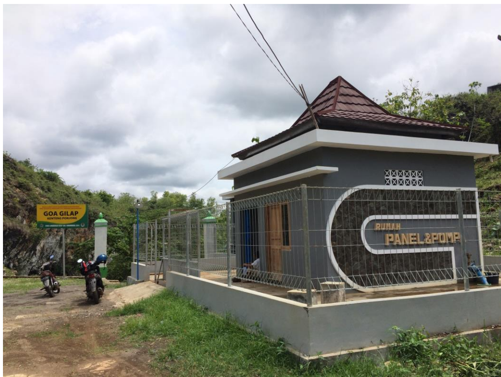
Gambar 4.15 Rumah Panel & Pompa di SPAM Songgilap
