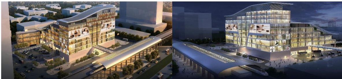
Gambar 2.16 Beijing Changyang Station TOD
