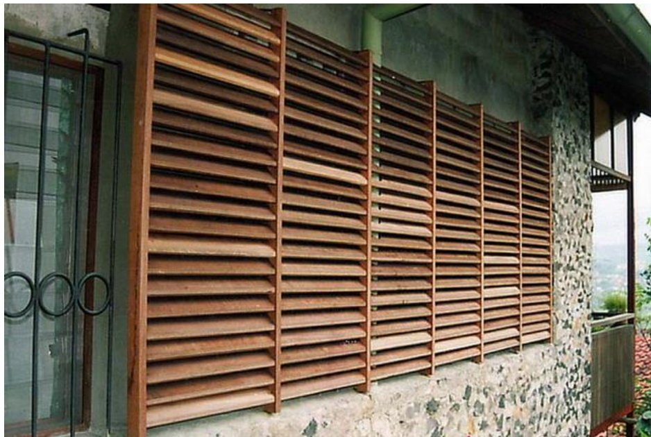
Gambar 2. 45 Sirap Bangunan Rumah Heinz Frick Sumber: https://archnet.org/sites/5066/media_contents/38718
