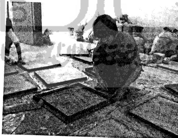
**Gambar 12.** Pelepasan Bekisting Sampel
