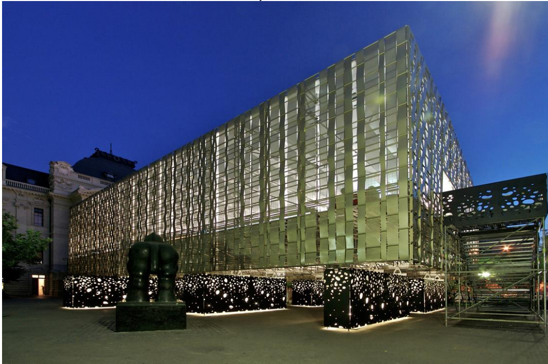
Gambar2.0.35 Pavillion XVI Chilean Architecture Biennale / Assadi + Pulido (Sumber: Archdaily-XVI Chilean Architecture Biennale,2018)
