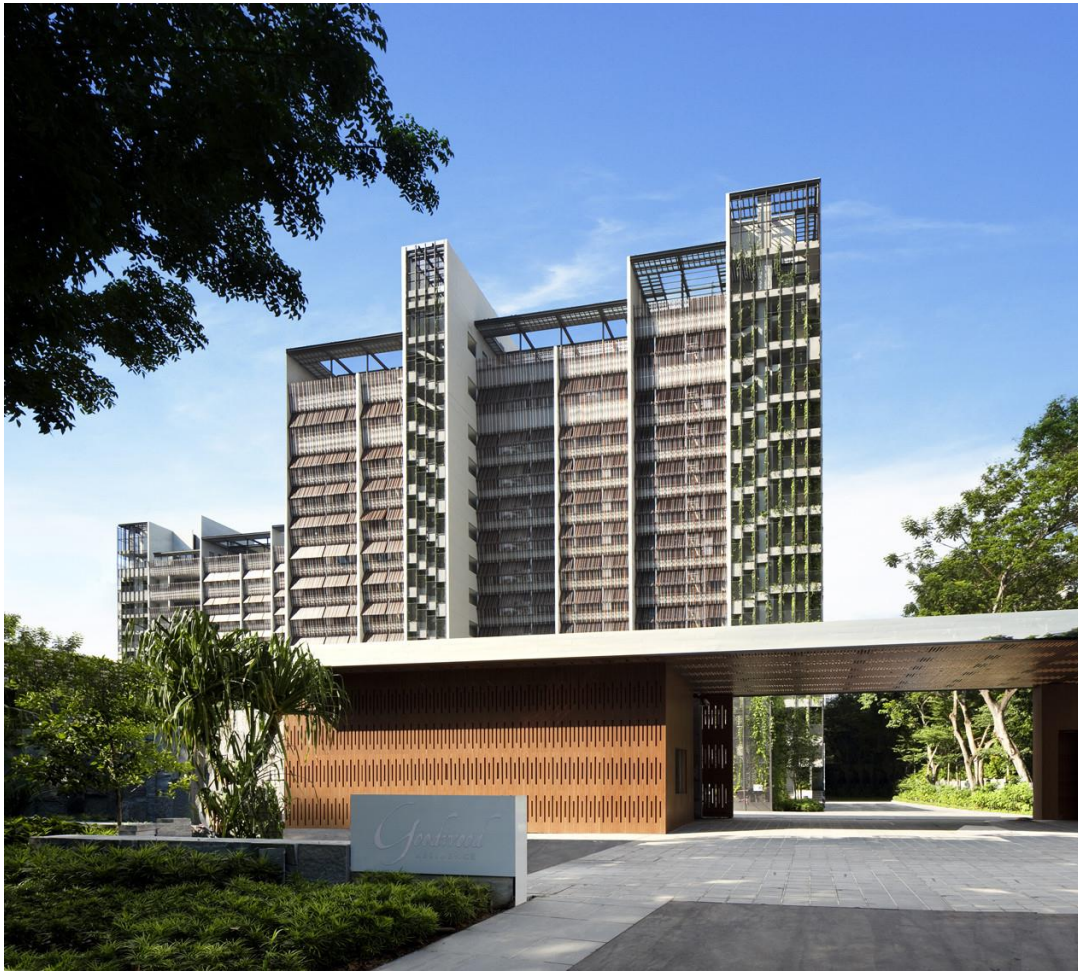
Gambar 2.3.2 Goodwood Residence Sumber : Archdaily. 2013
