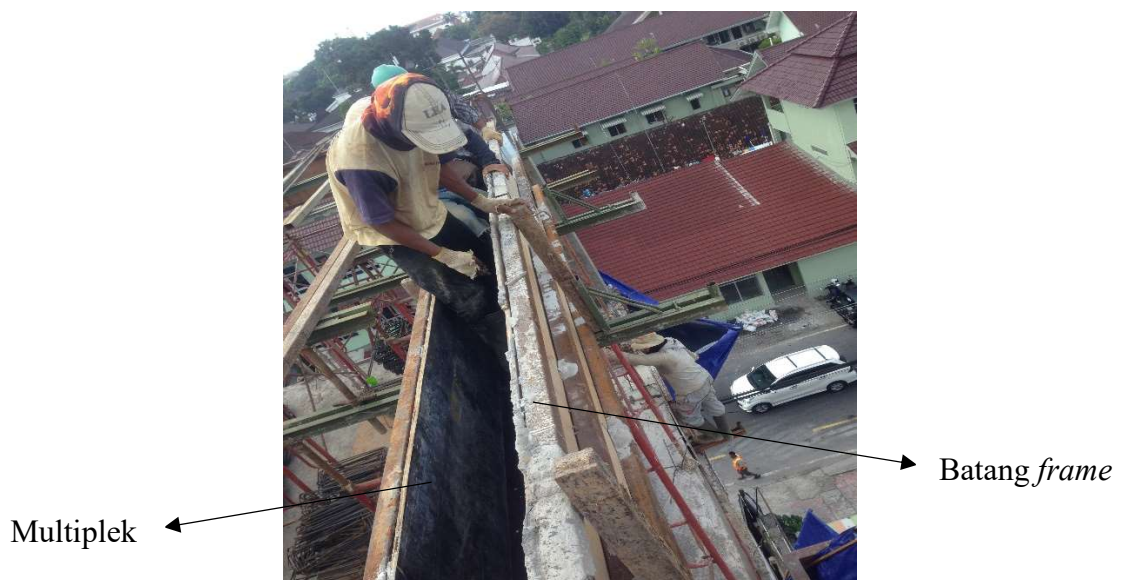
Gambar 5.4 Bagian-bagian Bekisting Balok
