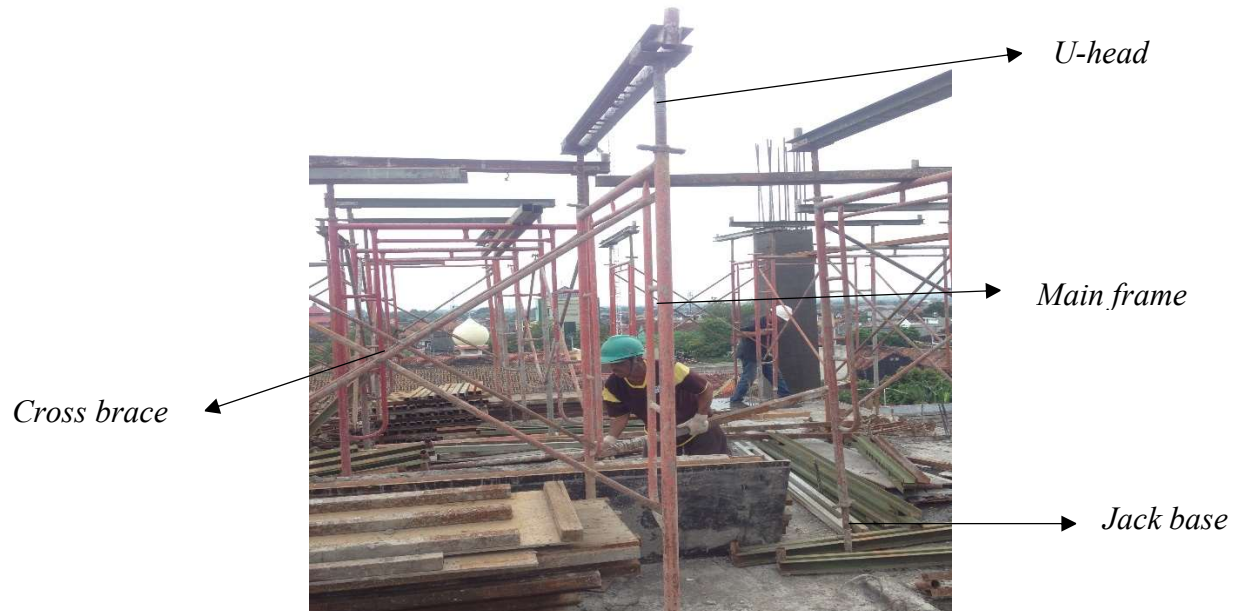
Gambar 5.5 Bagian-bagian Scaffolding
