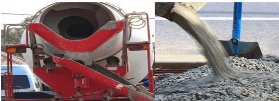
Gambar 4.4 Beton Ready Mix
