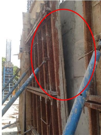
**Gambar 5.6 Bekisting Tidak Mampu Menahan Beton**
