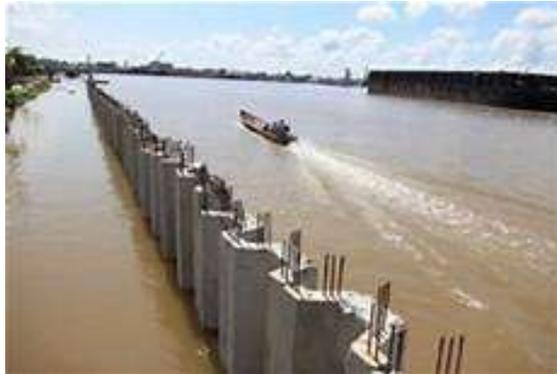
**Gambar 3.16 Sheet Pile Beton**
