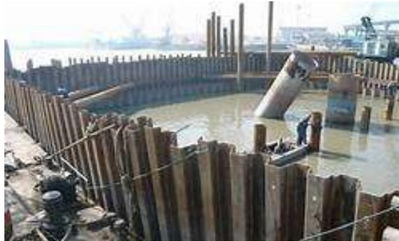
**Gambar 3.17 Sheet Pile Baja**
