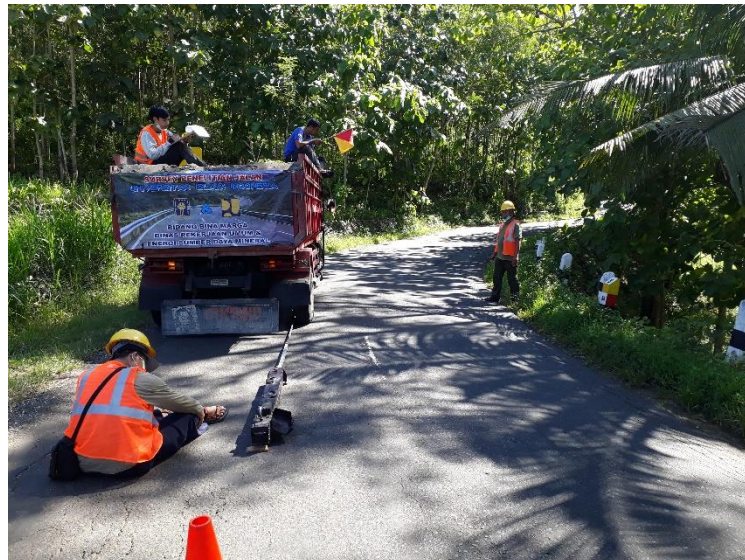
Gambar L-4.7 Uji Lendutan Balik ( Benkelman Beam )
