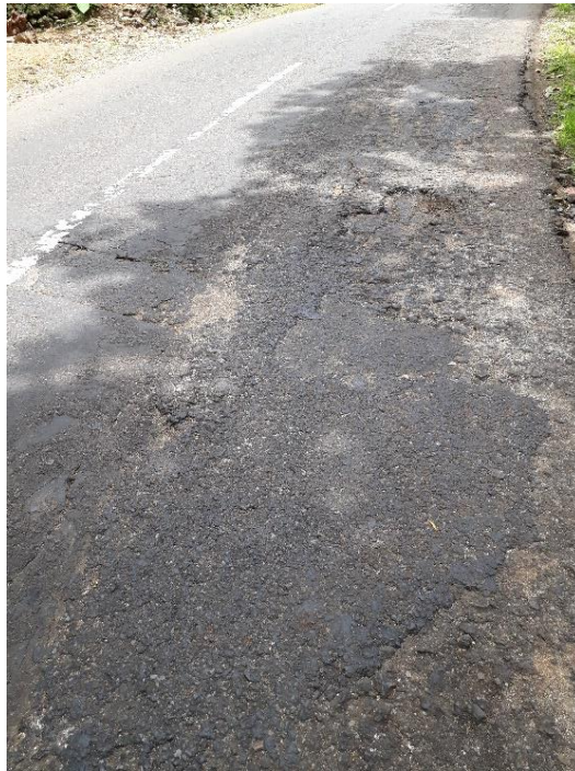
Gambar 1.3 Pelapukan dan Butiran Lepas ( Weathering and Raveling )
