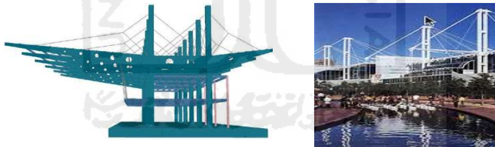
Gambar 2.16. System struktur kabel (Sumber: http://spacetrussbuilding.blogspot.com , 2015)
