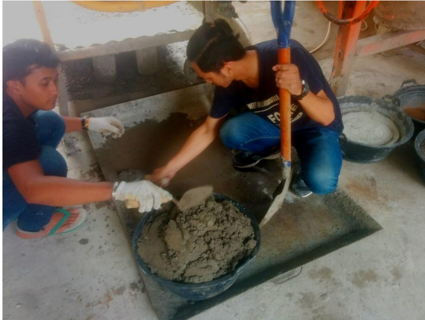
Gambar L-2.1 Proses Mixing Mortar Papercrete
