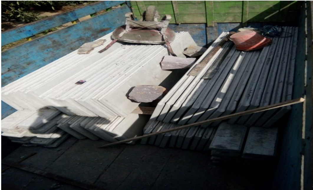
Gambar L 4.1 Bahan Material Pagar Beton Precast
