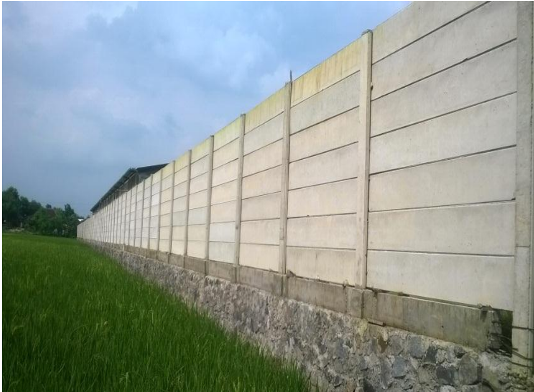
Gambar 3.1 Pagar Beton Precast Sistem Knock Down (Sumber: PT. Powercon Jaya Utama)
