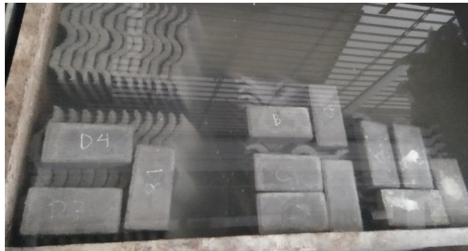
Gambar 4.22 Proses Perawatan Paving Block
