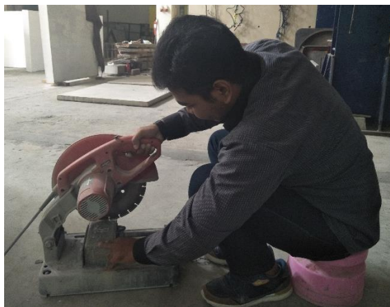
Gambar 4.23 Proses Pemotongan Paving Block
