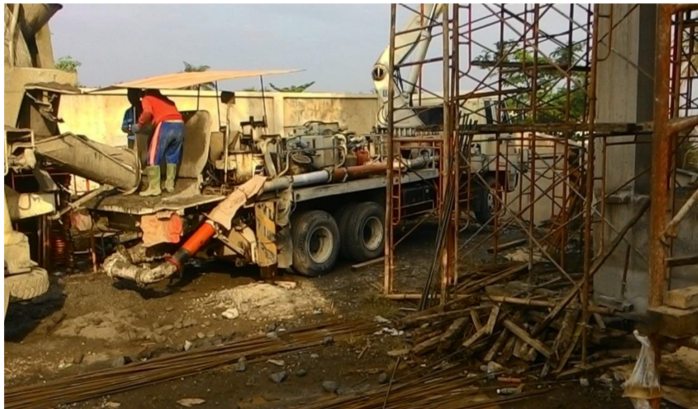
Gambar L 3.2 Concrete Pump Truck
