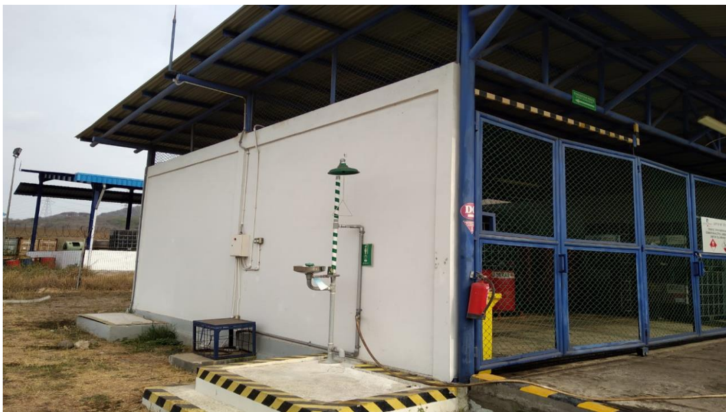
Gambar 4.3 Gedung Shelter at Ash Disposal
