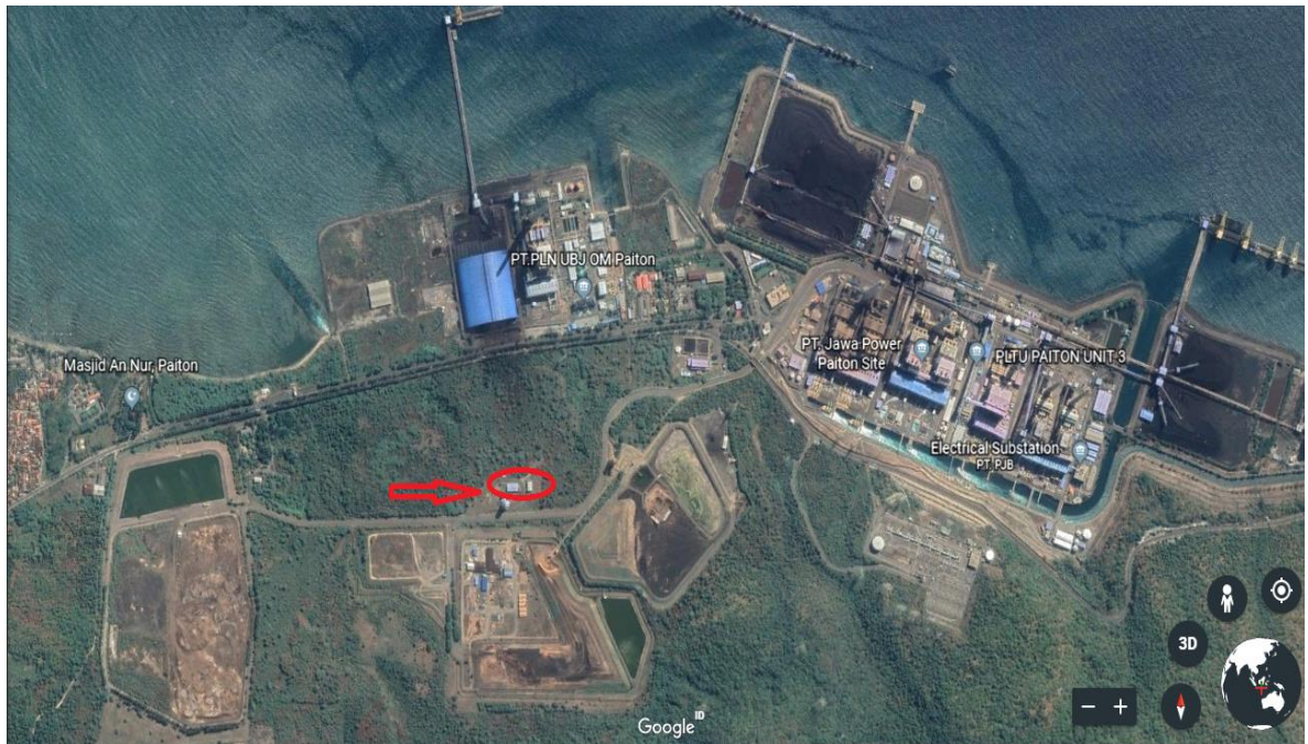
Gambar 4.1 Lokasi Proyek Shelter at Ash Disposal Sumber : https://www.earth.google.com
