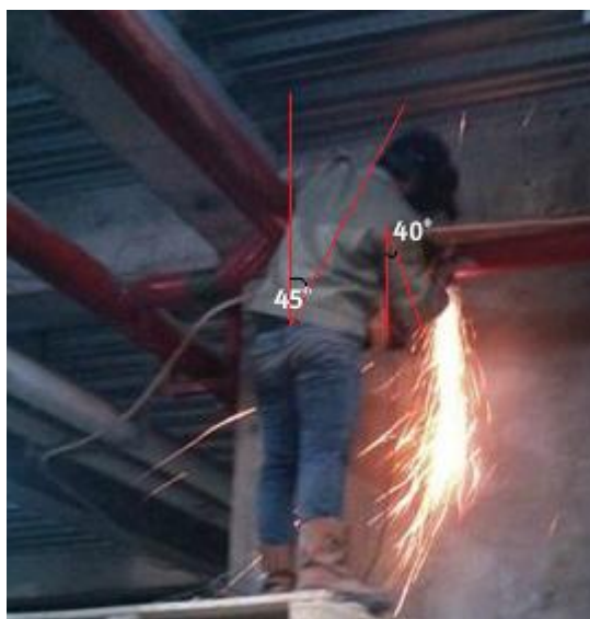
Gambar 4.5 Proses penghalusan pipa besi
