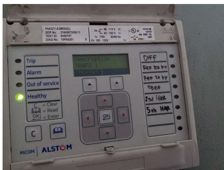
Gambar 2.1 Relay Differensial GI Cilegon Lama
