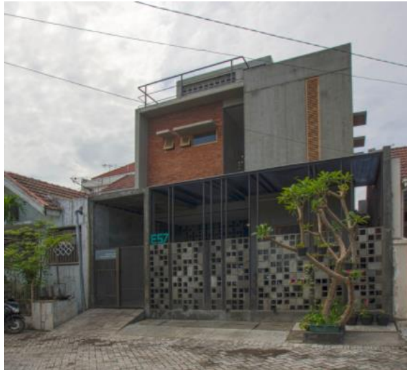
Gambar 2.32 Boarding House di Surabaya
