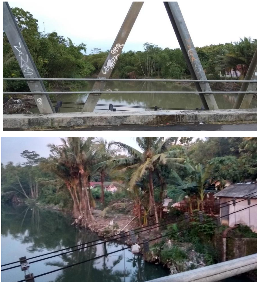
Gambar 3.9 Site 3 (Jembatan Blawong)
