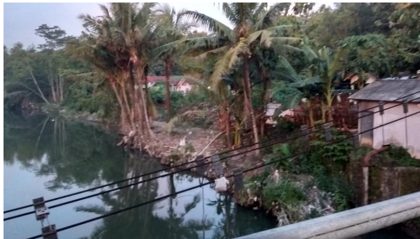
Gambar 3.10 Site 3 (Jembatan Blawong)
