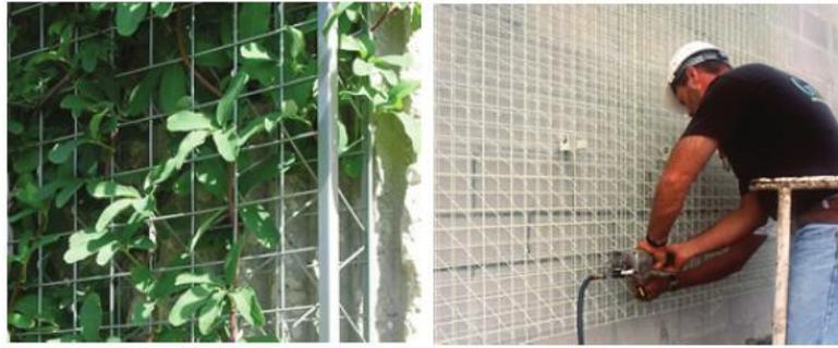
*Gambar 2 20 Tipe Modular trellis panel system*
