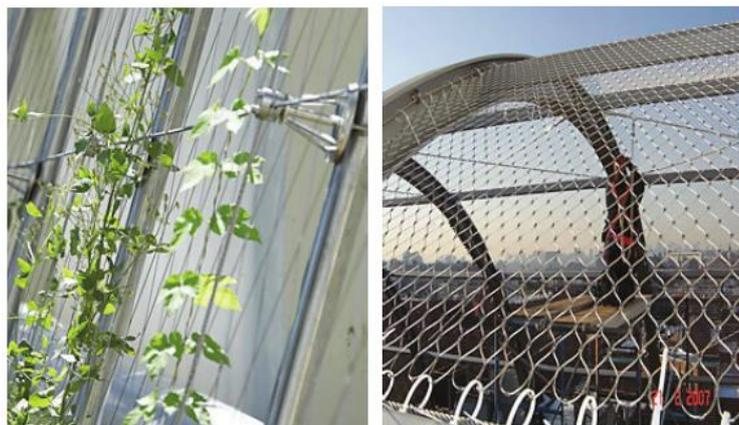
*Gambar 2 21 Tipe Wire rope net system*
