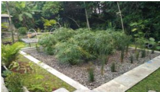
**Gambar 2.2**Horizontal Gravel Filter
