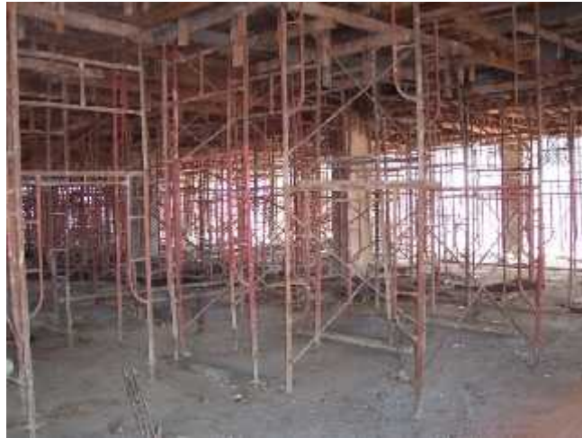
Gambar 3.3 Pemasangan Perancah ( Scaffolding )
