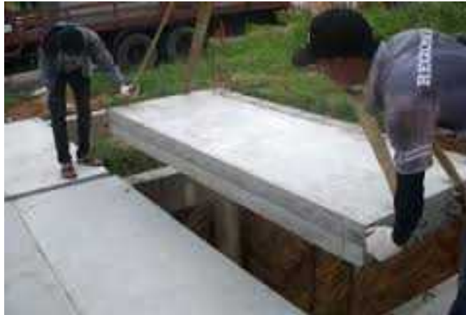
Gambar 3.6 Proses Erection
