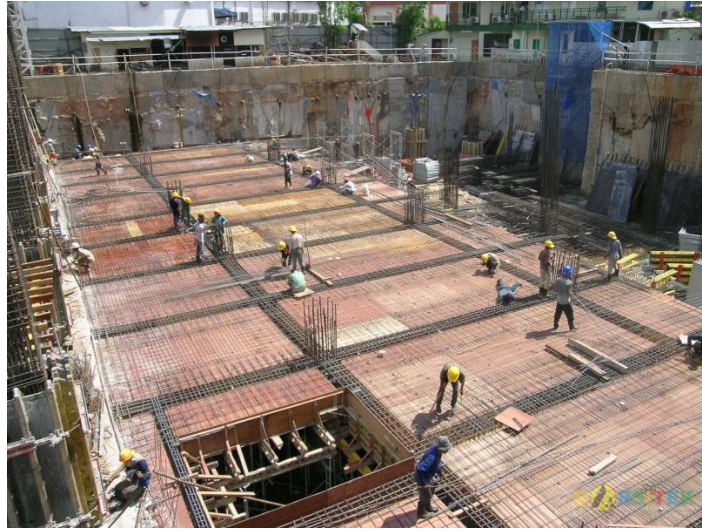
Gambar 3.4 Bekisting (Sumber: www.cyrilengineering.blogspot.co.id )
