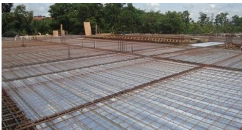
Gambar 3.6 Pelat Lantai Steel Deck (Sumber: www.rian-desti.blogspot.co.id )
