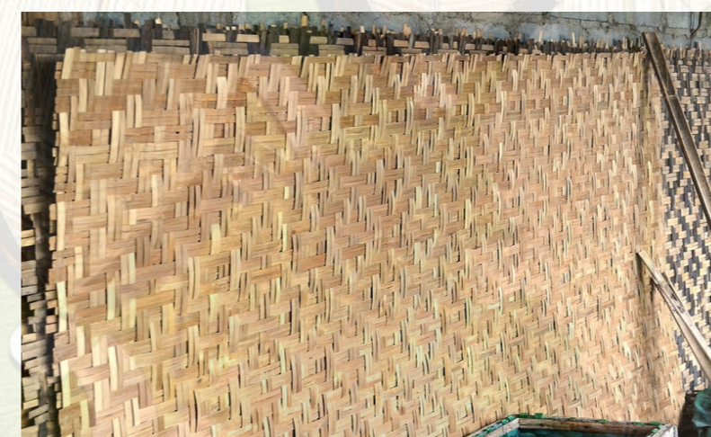
DINDING ANYAMAN BAMBU] (GEDHEG)
