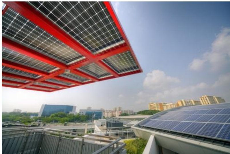
Gambar 2.14 Penerapan Shading Devices
