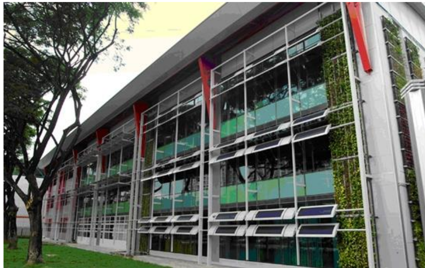
Gambar 2.12 Penerapan Shading Devices
