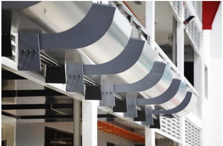
Gambar 2.11 Penerapan Mirror Duct
