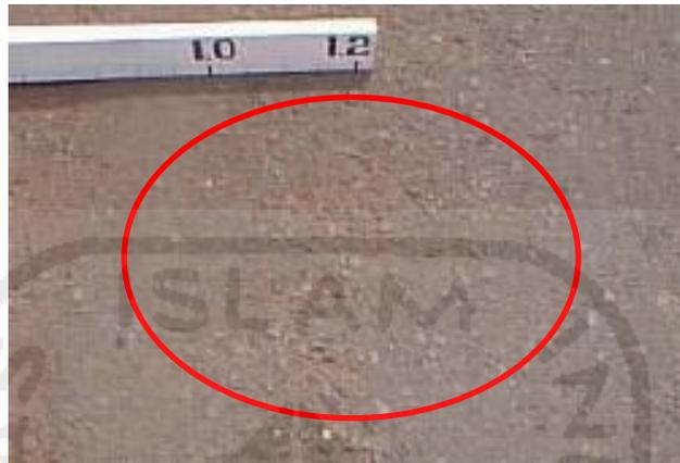
Gambar 3.14 Agregat Licin (*Polished Aggregate*)
