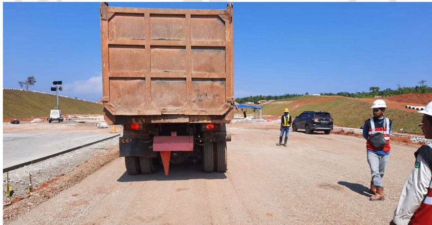
Gambar 73. Uji Profrolling Top Subgrade
