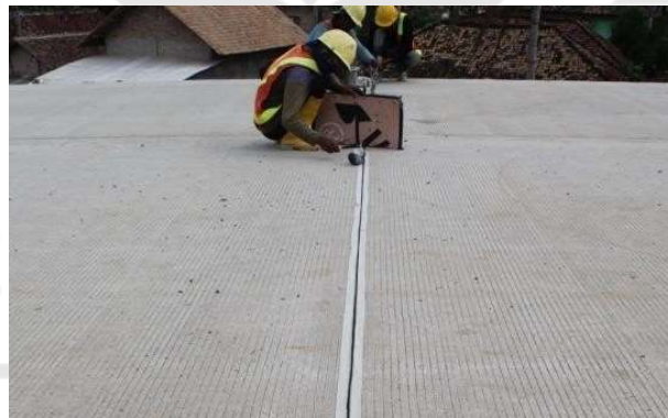
Gambar 37. Pekerjaan Joint Sealant
