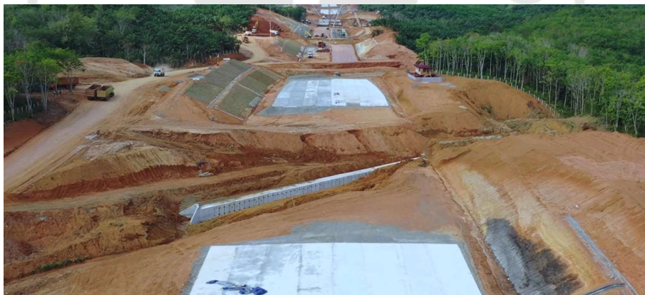
Gambar 64. Pekerjaan Lean Concrete Terpotong Box Culvert
