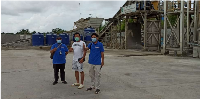
Gambar 79. Batching Plant PT. Super Beton Prima
