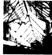
Center mall skylight
