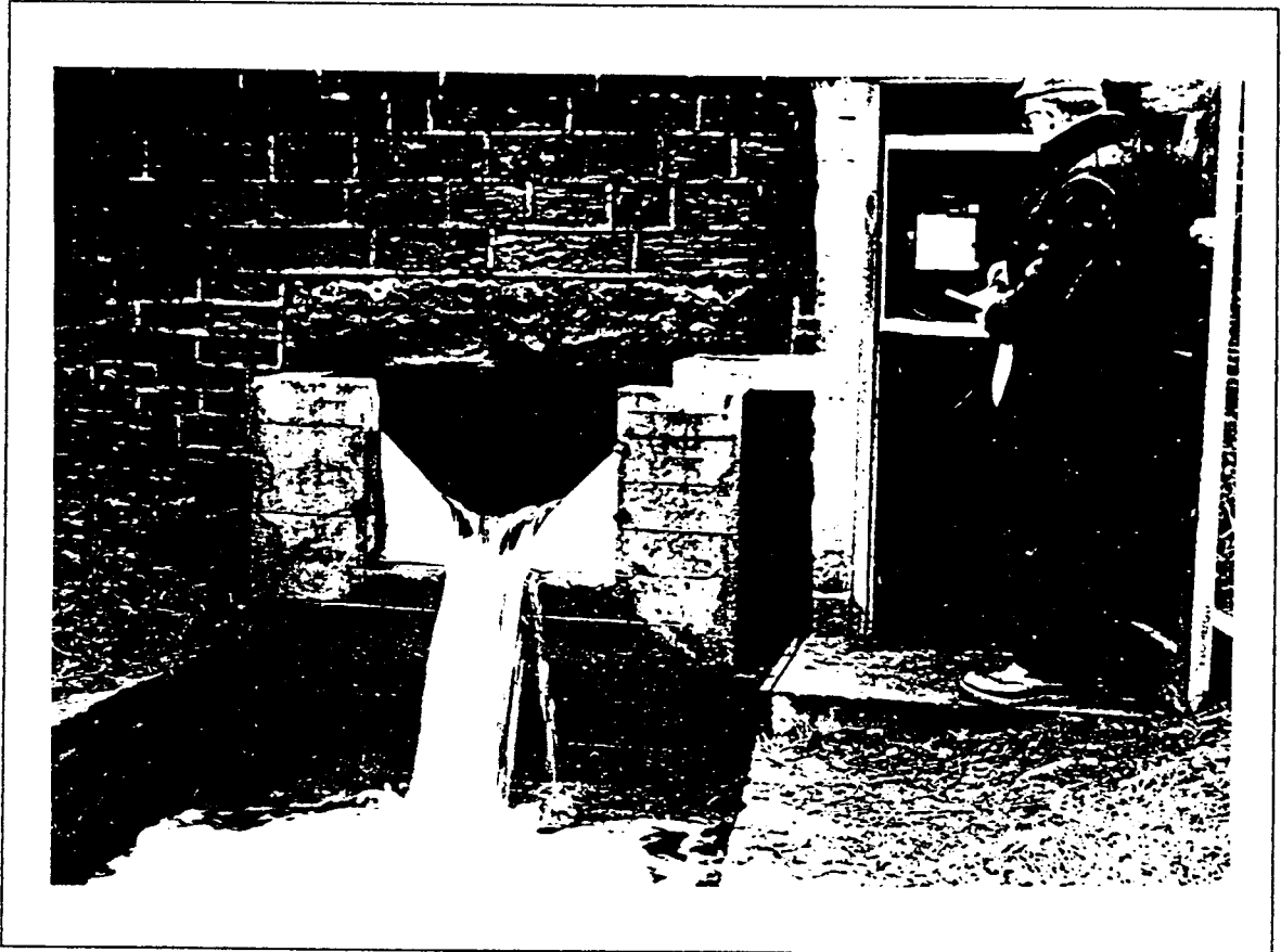
Gambar bendung "v-notch"
